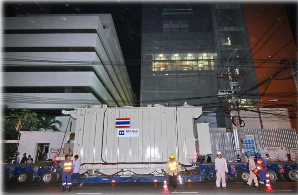
300 MVA 220 – 69 – 24 kV Metropolitan Electricity Authority Chidlom Terminal Station, Bangkok THAILAND
